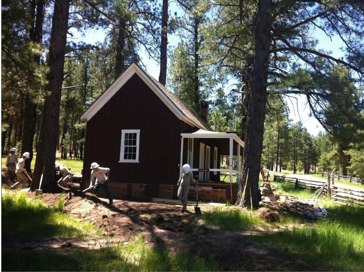
ACE crew cleans out and expands drainage ditches during the Jacob Lake Ranger Station cabin restoration project, June 2016. Photo by Connie Reid. Credit the U.S. Forest Service, Southwestern Region, Kaibab National Forest.
