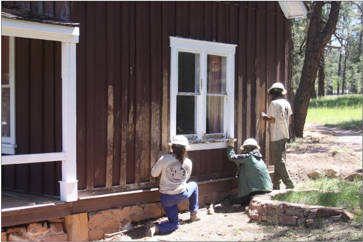
ACE crew scrapes loose paint prior to repainting, June 2016. Photo by David Hercher. Credit the U.S. Forest Service, Southwestern Region, Kaibab National Forest.
